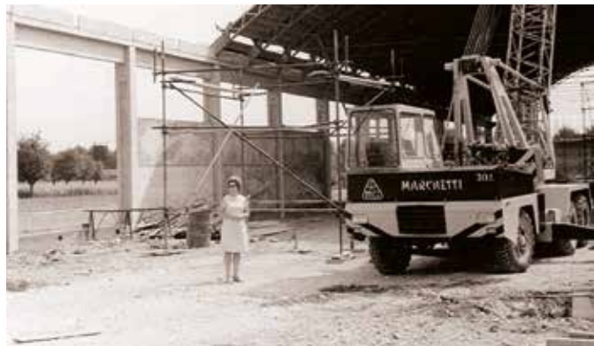
Mrs. Donella Nesti supervising the construction of the new factory May, 1970
